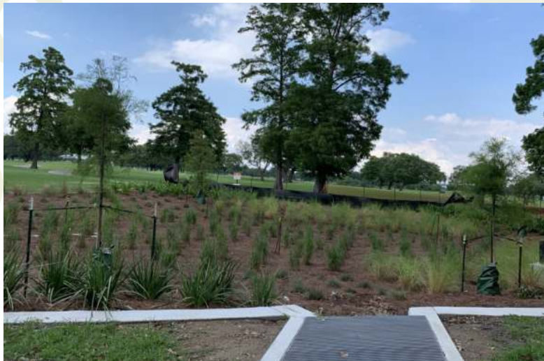
Near-complete stormwater detention basin - PONTILLY
