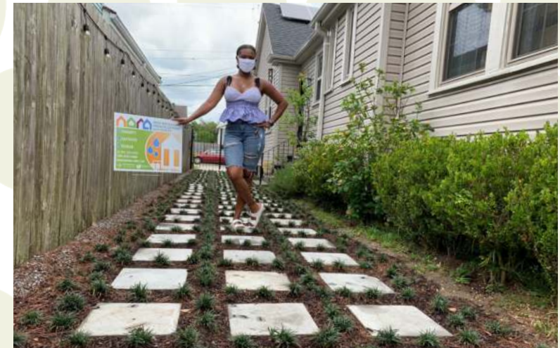
Community Adaptation Program participant with newly installed infiltration trench - GENTILLY
